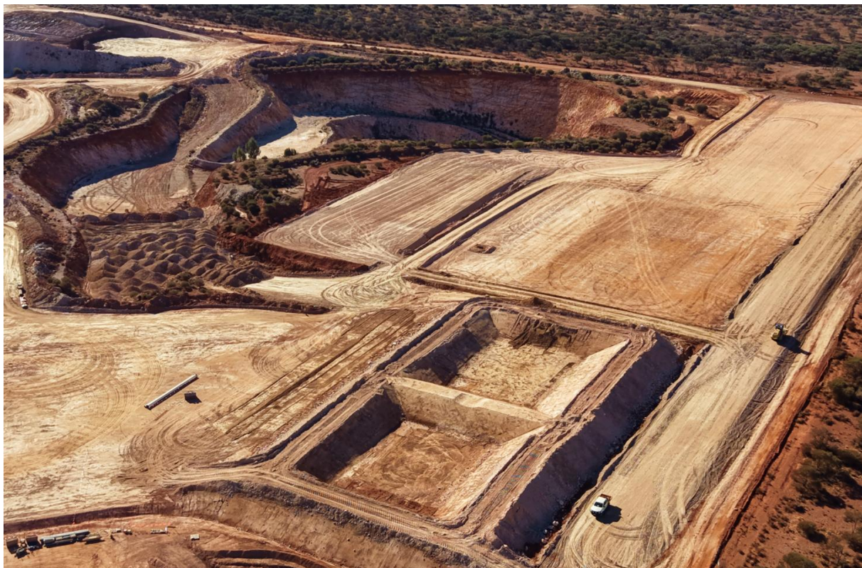
Figure 7: Raw and Process Water Ponds and Earthworks Pads (July 2026)
