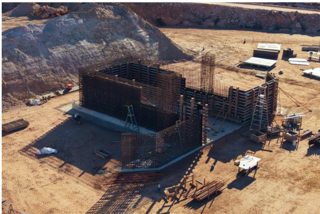
Figure 3: Primary Crusher Wall and Foundations (July 2026)
