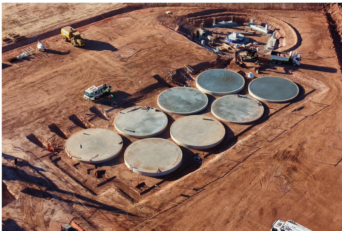
Figure 6: CIL tank footings (July 2026)
