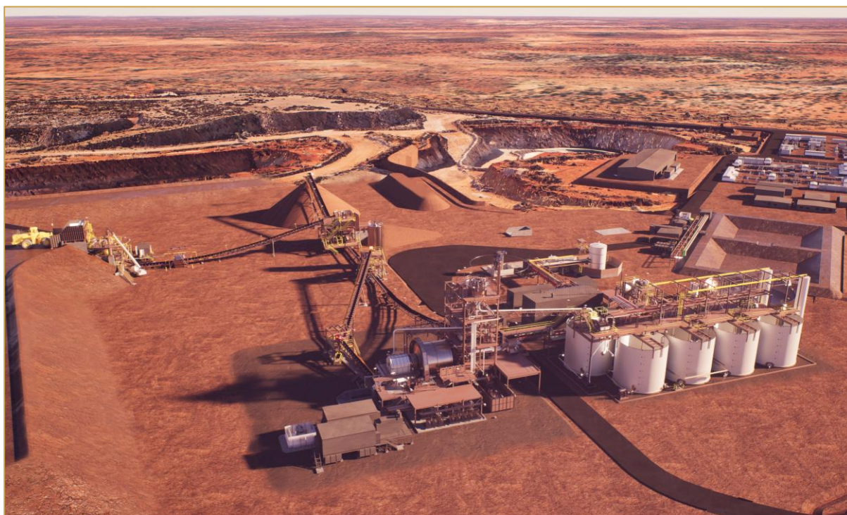
Figure 1: Laverton Processing Plant - 1.5Mtpa design render
