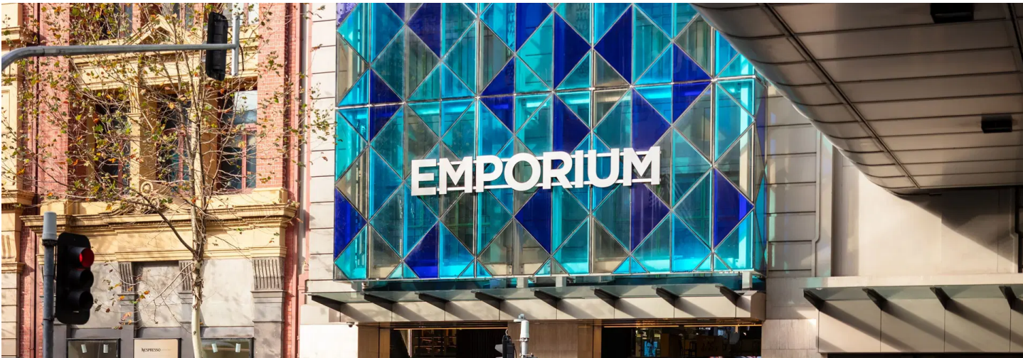
Emporium Melbourne, VIC Credit: Vicinity Centres
