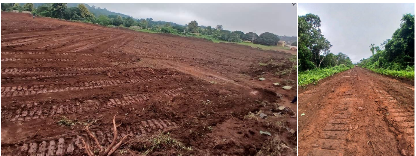
Figure 6 Bondoukou. Clearing designated parcel of land and road repairs for the Dingbi Village community within the Bondoukou Project area.
