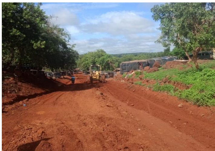
Road Upgrade in Kobada Village
