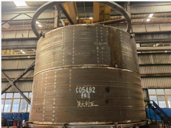
Ball mill shell construction
