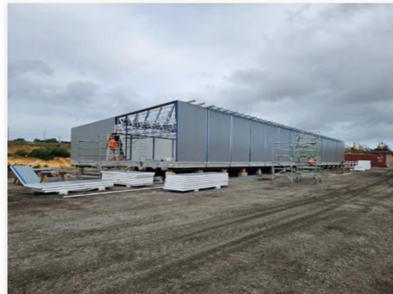
Permanent MSA 1 building construction
