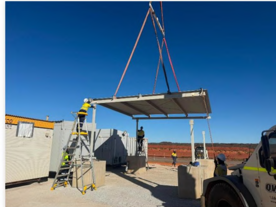
Project offices on-site works
