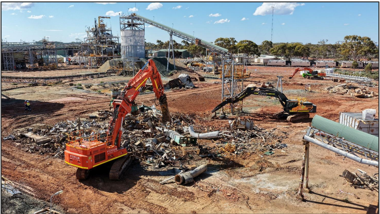
Figure 1 – Demolition of redundant conveyors and structures
