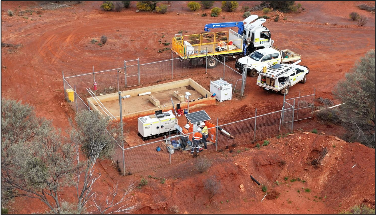
Figure 3 – Borefield refurbishments in progress
