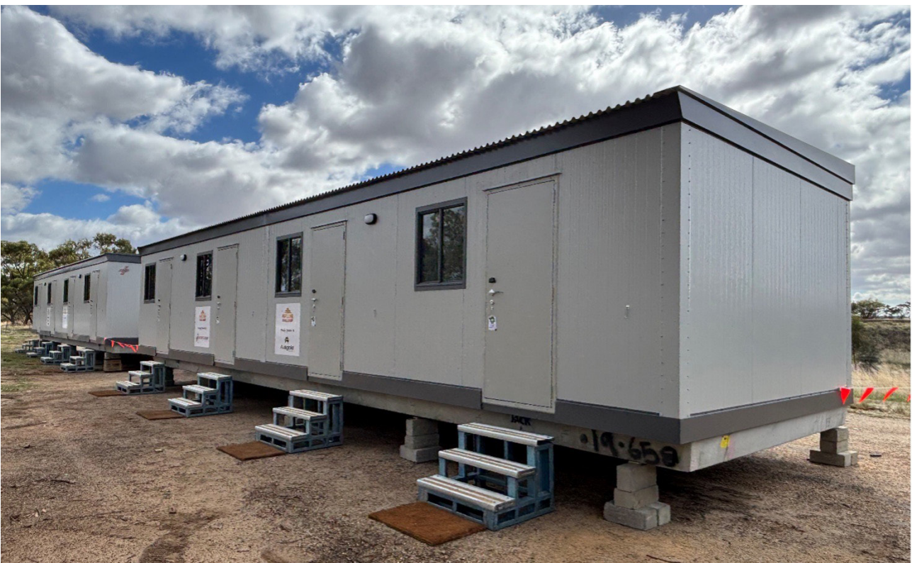
Figure 2: Prefabricated Workforce Accommodation Facility modules
