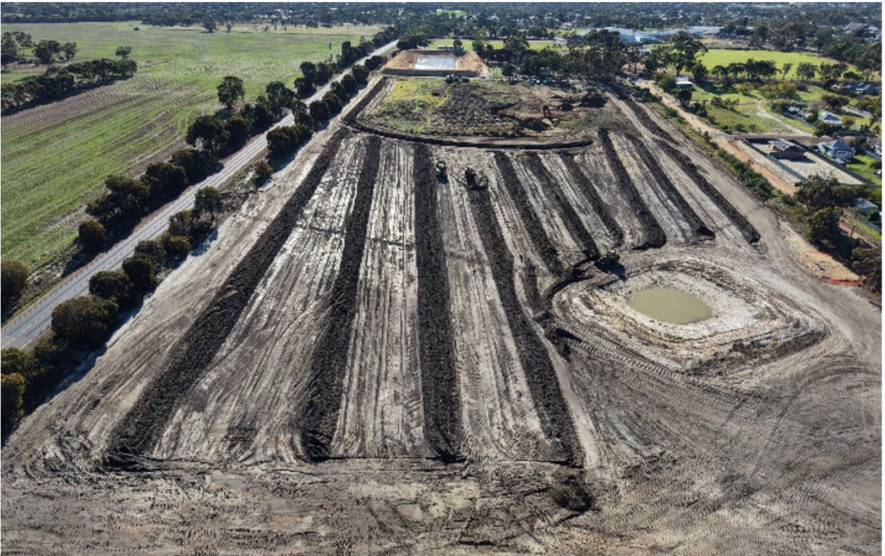
Figure 1: Workforce Accommodation Facility under development
