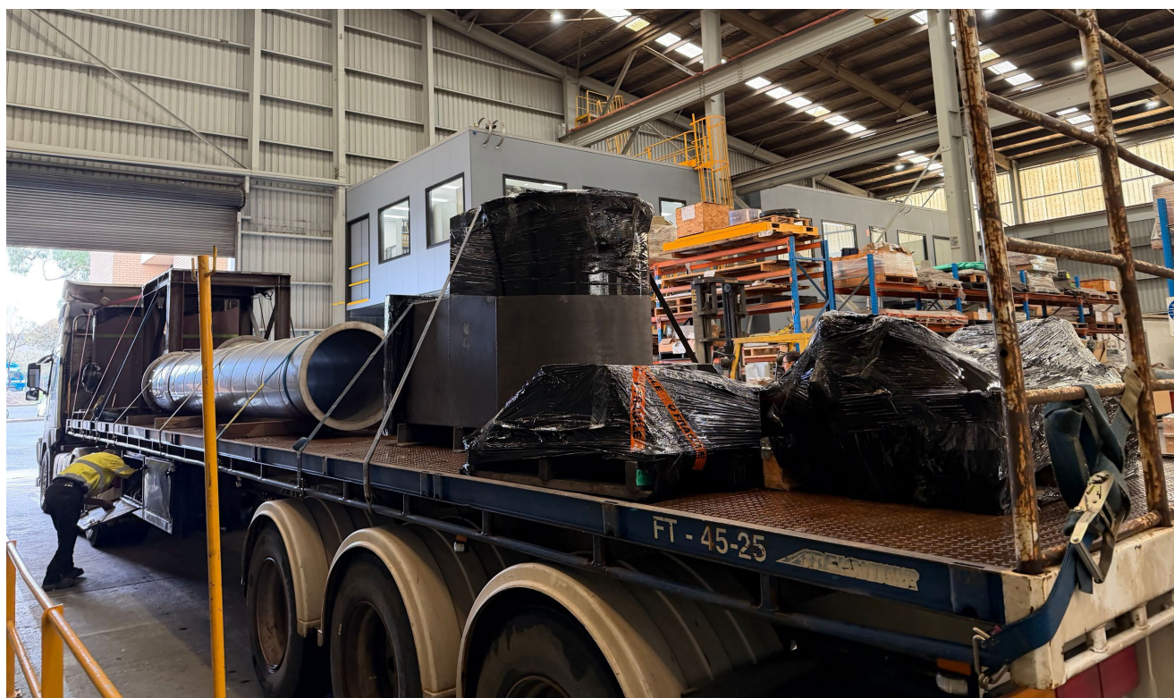
Delivery of last remaining outstanding equipment, including exhaust stack and combustion gas piping
