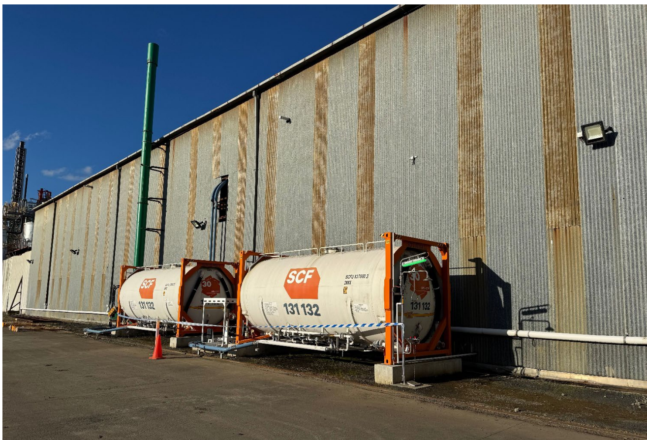
Briquetting (top) & Quicklime (bottom) area installation completed and ready for staged commissioning and testing
