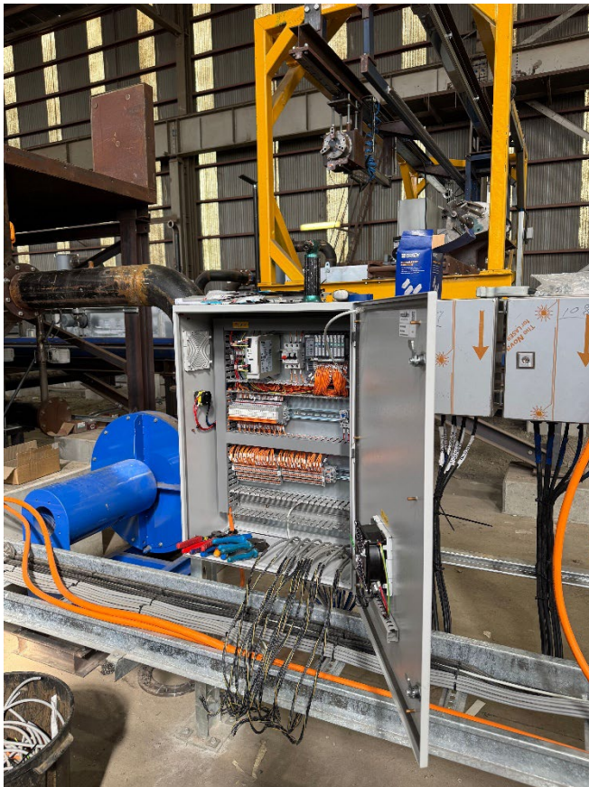
Reduction Furnace area electrical and instrumentation cable installations for the furnace, automatic shuttles and baler equipment control panels and field junction boxes progressing
