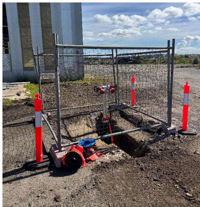
Fire protection installation with fire hose reels completed and new hydrants progressing
