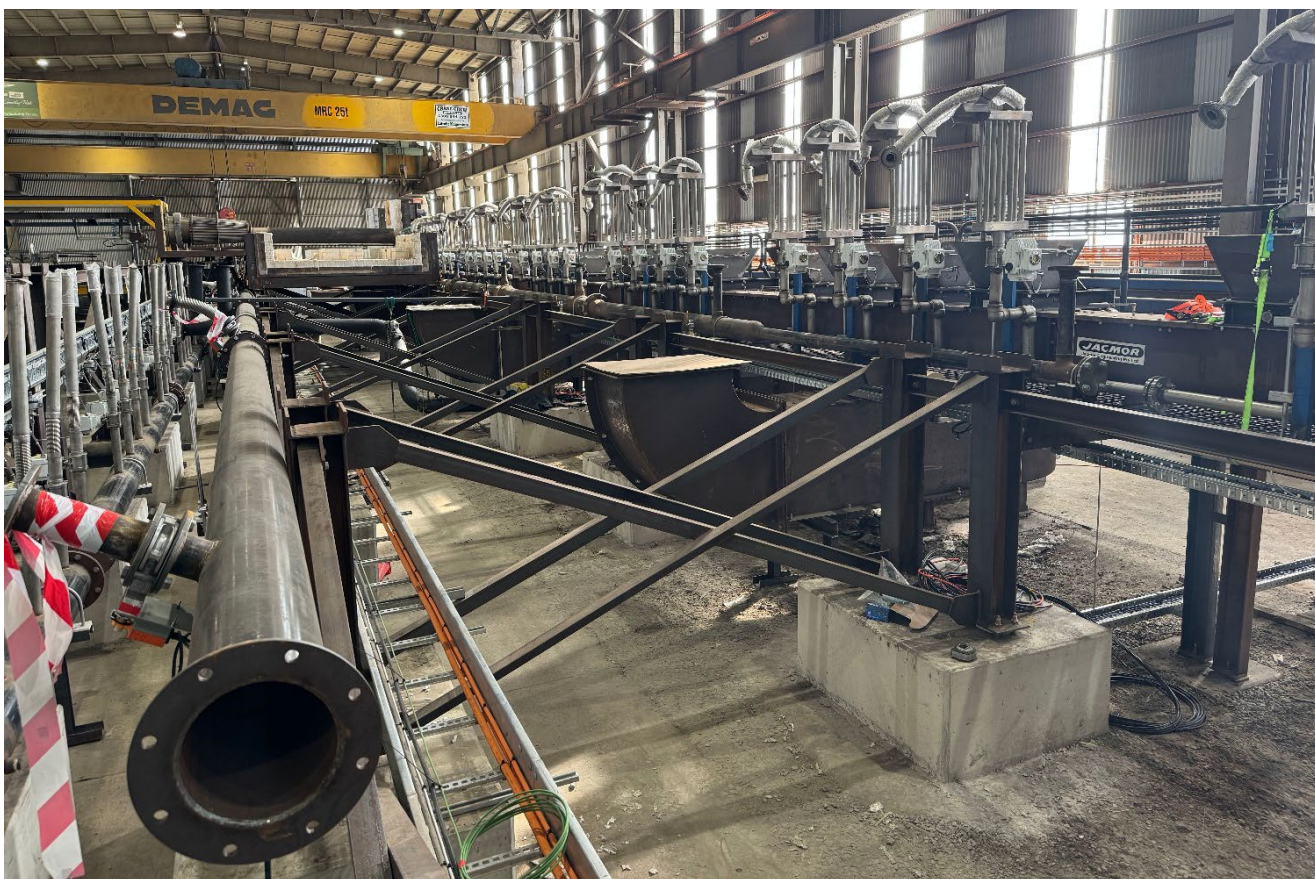
Reduction Furnace area installation progressing with exhaust ducting, air aspiration piping, and bottom modules with burner controls
