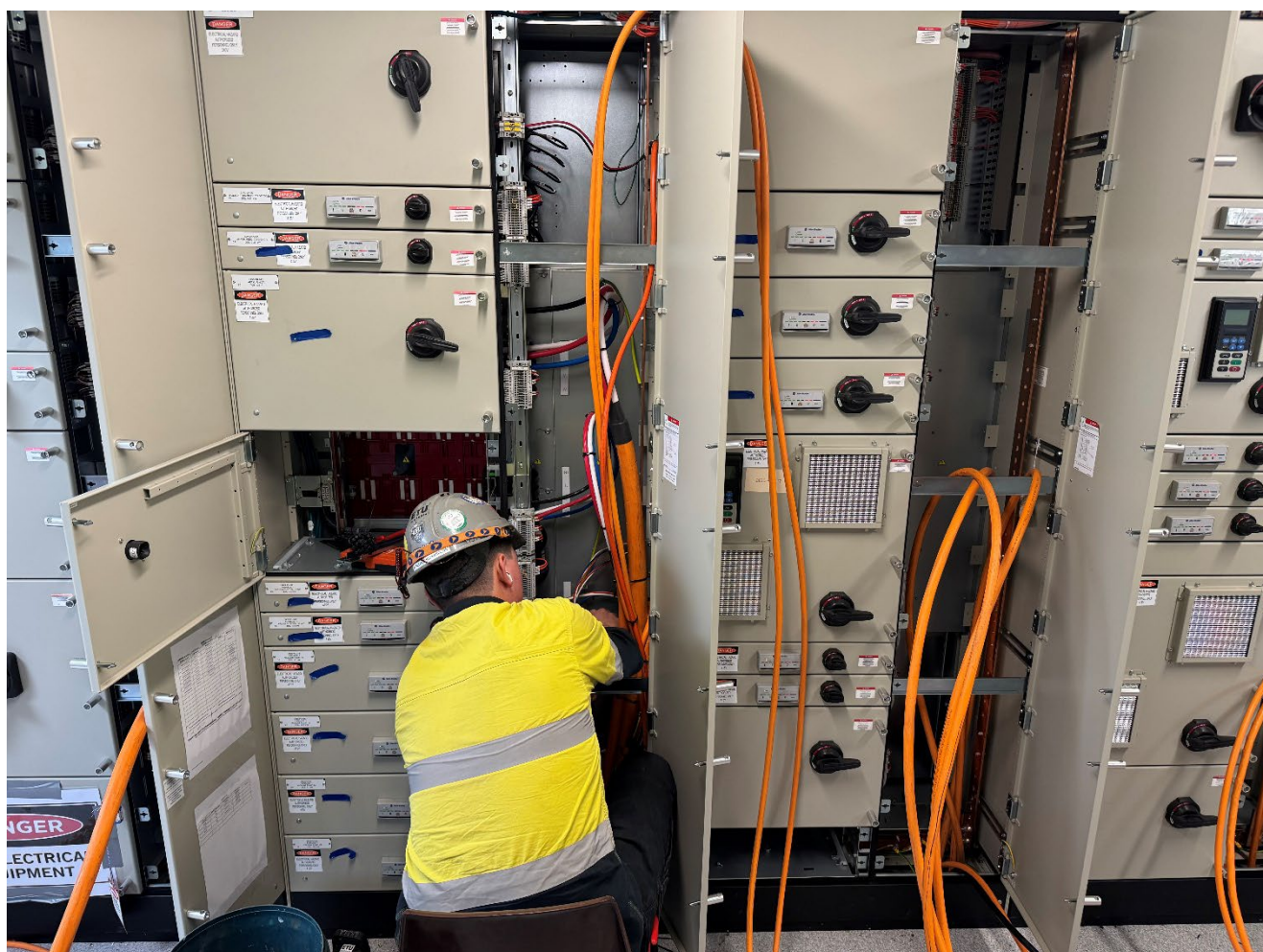
E&I electricians progressing with terminations within the substation for Reduction Furnace area equipment
