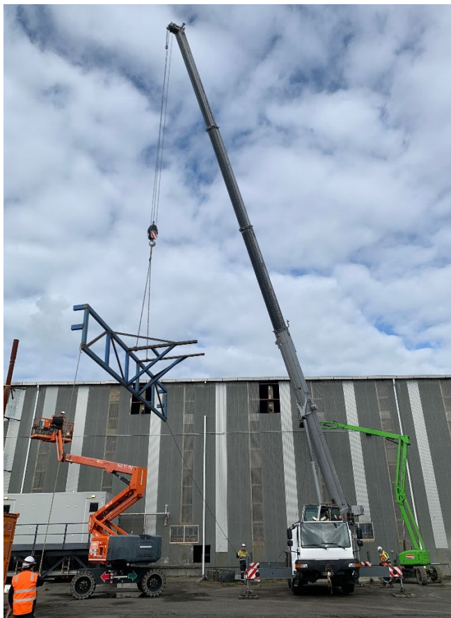
Briquette Loading Storage Hopper safety cages, Reduction Furnace stack support and piping installation progress
