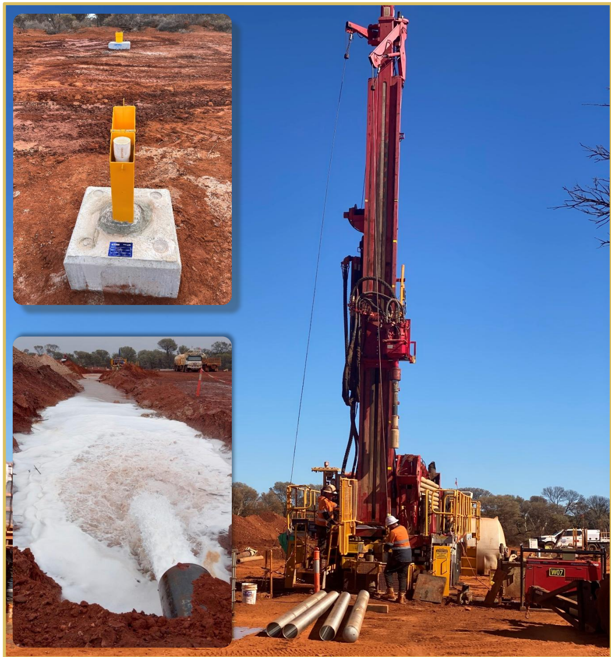
Figure 5 – Installation of screen for water production bore at Lake Raeside Paleochannel. Inset showing completed production bore and monitoring bore (inset top left), and ~30 L/s air lift testing of completed production bore (inset bottom left)
