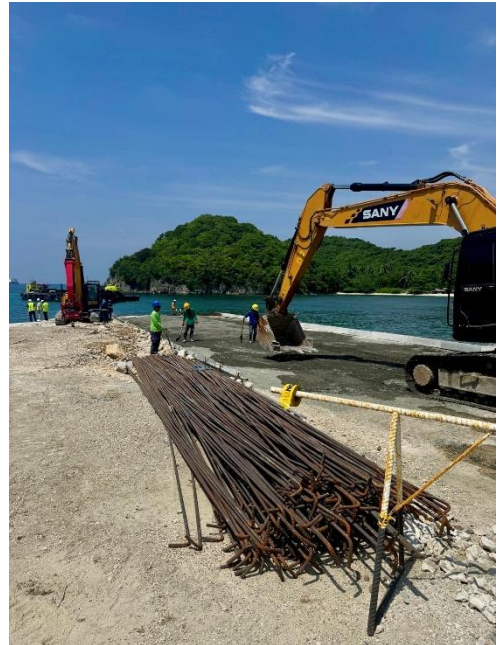
Site works supporting turbine loading and shipment preparations at Pagbilao, August 2026
