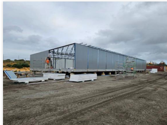
Permanent MSA 1 building construction
