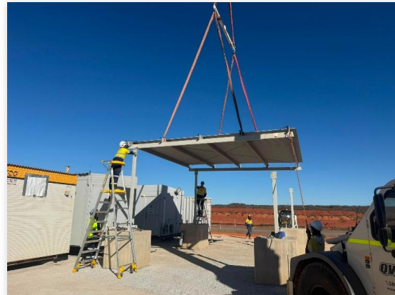
Project offices on-site works
