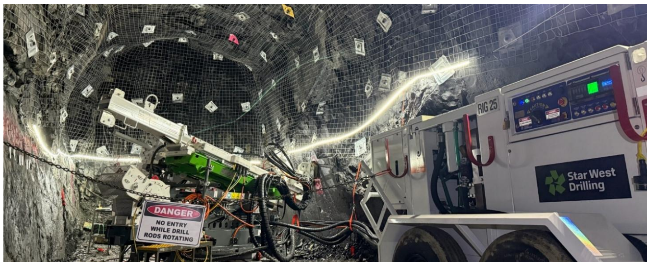
Figure 1. Drill rig at the face, Northern Drill Drive
