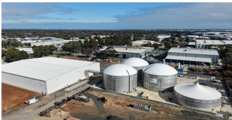
SA1 Salisbury Bioenergy construction
