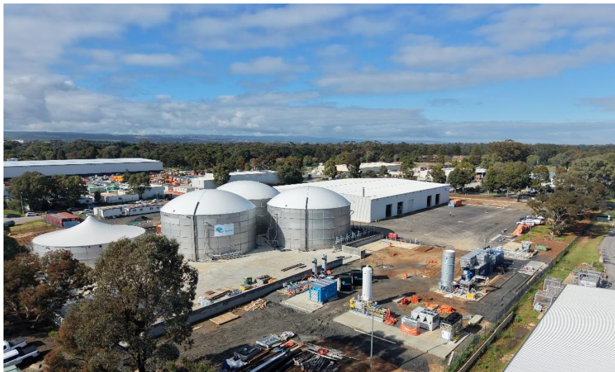
SA1 Salisbury Bioenergy construction
