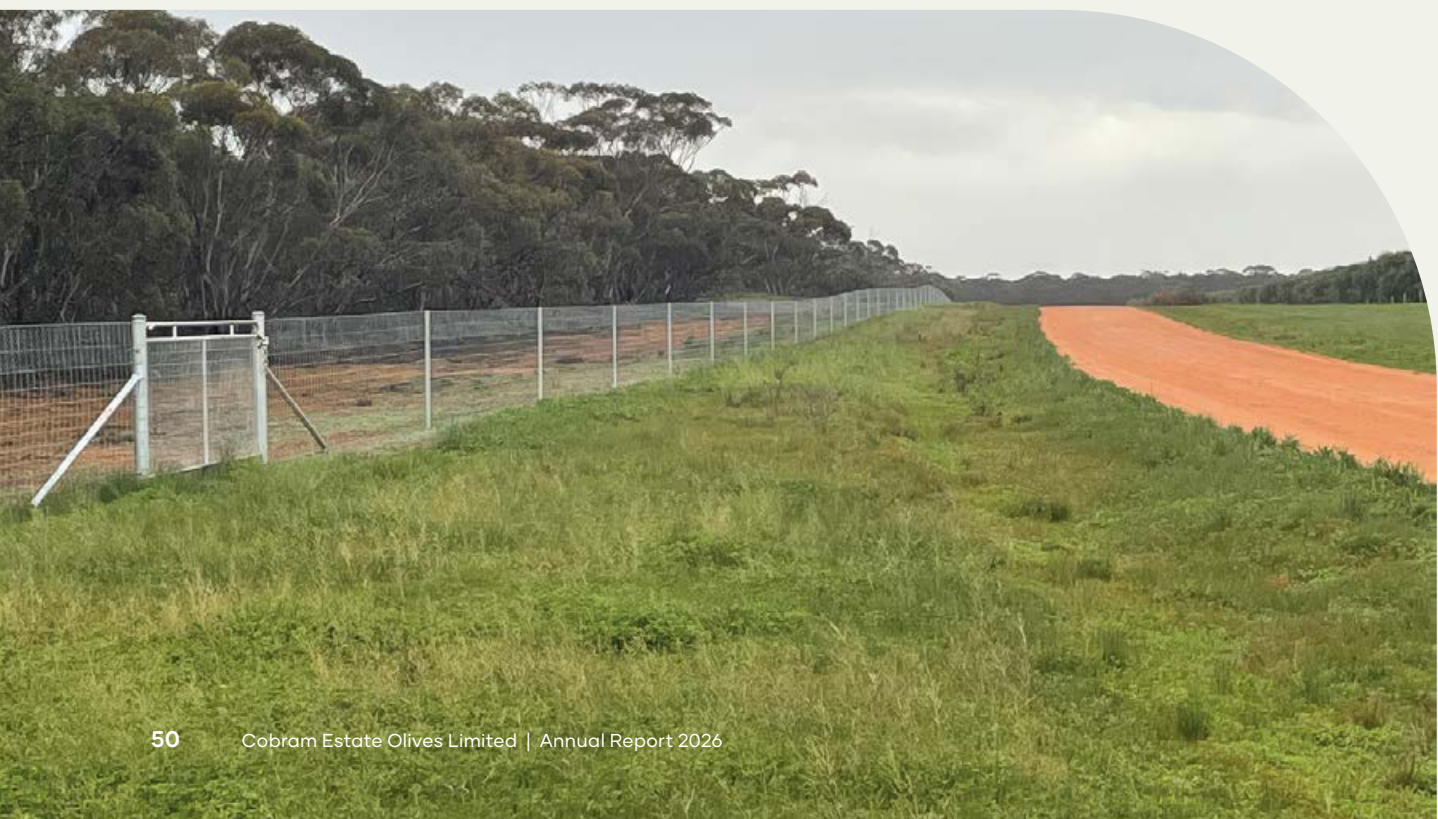
CONSERVATION EXCLUSION FENCE AT BOUNDARY BEND
