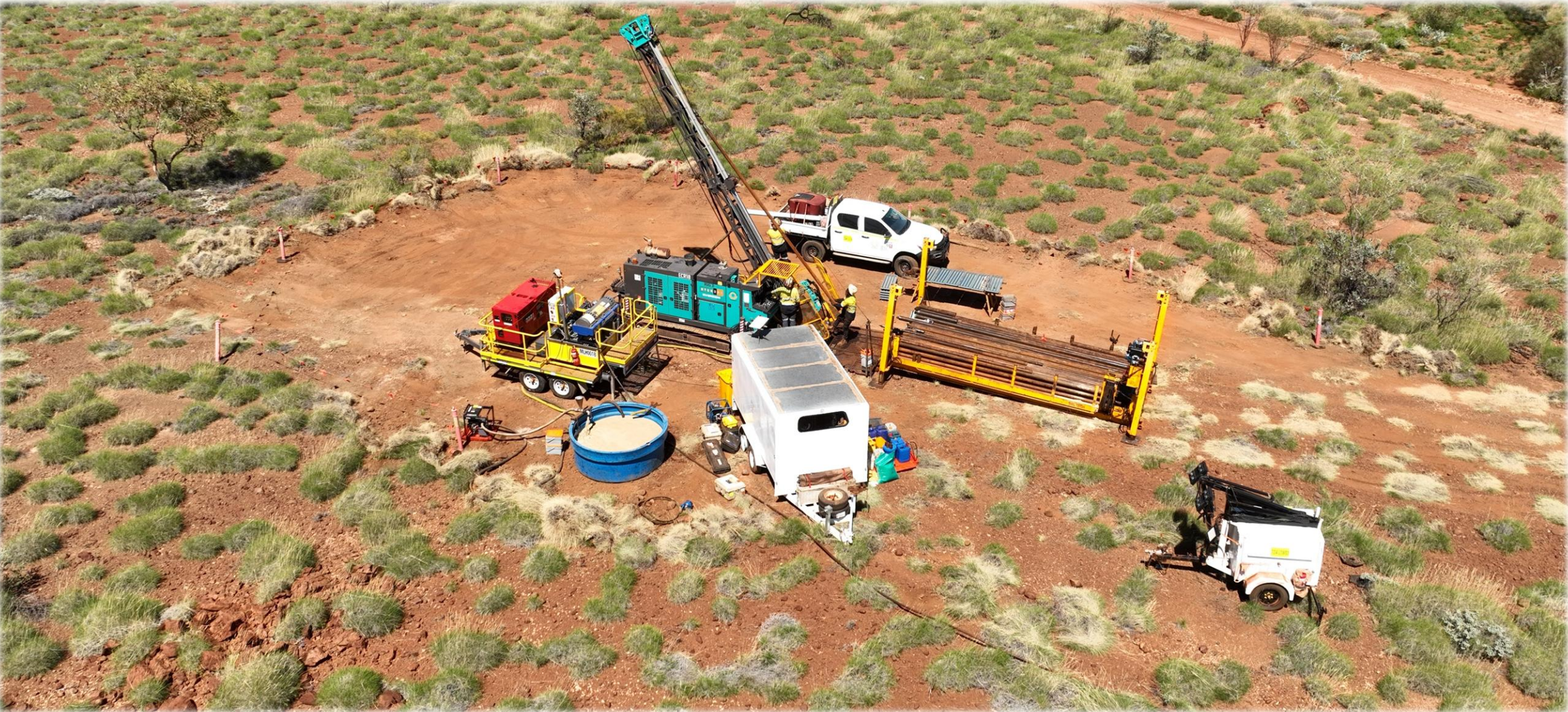
Drill Site Operations: Core drilling setup and ancillary equipment deployed on-site during the latest phase of resource expansion drilling at Elizabeth Hill.
