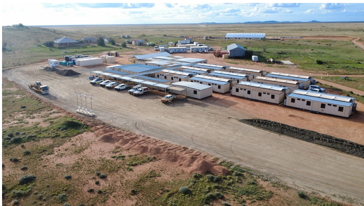
Figure 2 Sandfire's new 80-person onsite camp located adjacent to the Kalkaroo homestead and Havilah's long-term exploration camp. The new drillcore processing facility is under construction (white roof in the middle distance).
