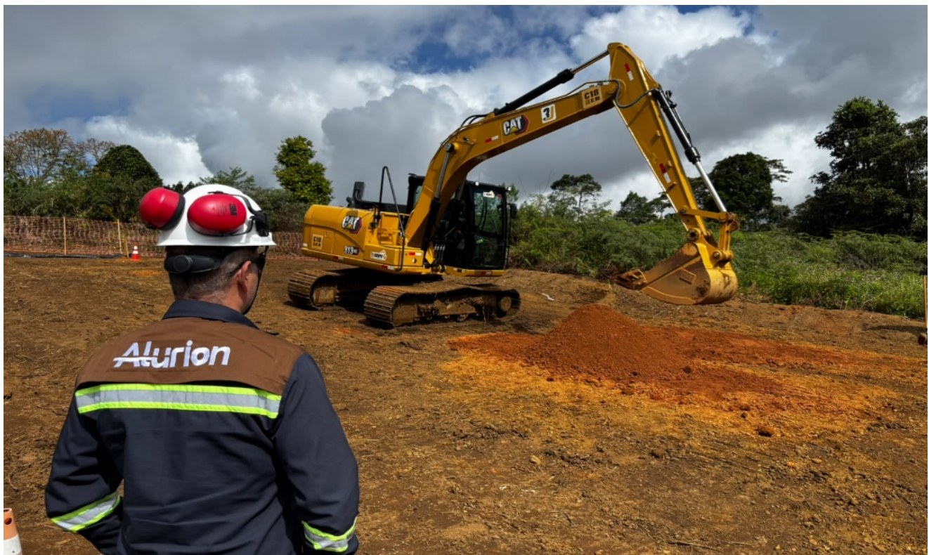
Figure 3: Alurion's first trench operation in Lapa target, site AMBX1951, Central District, Amargosa Project
