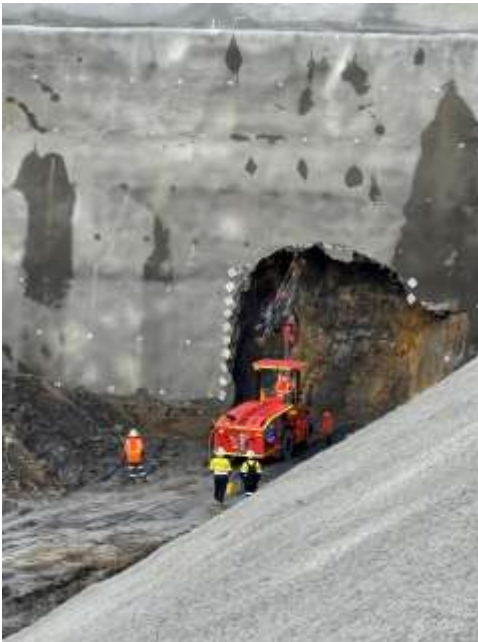
Figure 3. Scaling the first cut at the portal face.
