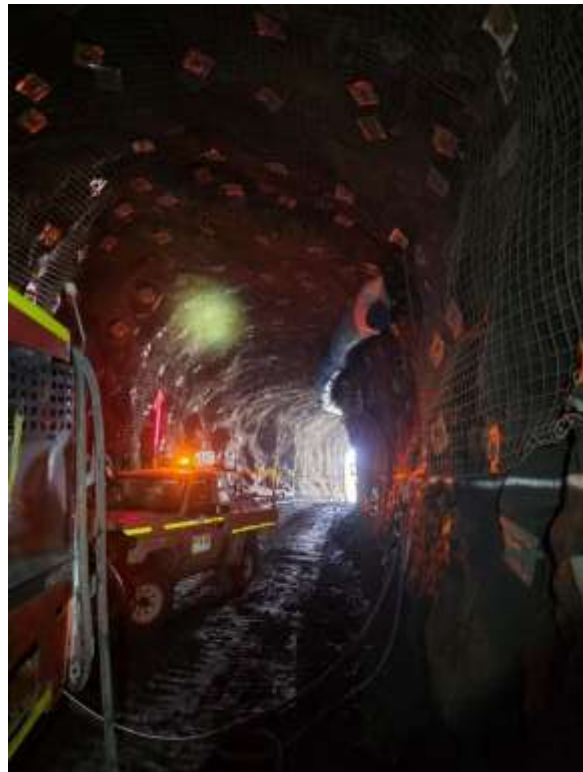
Figure 7. Exploration Decline development July 2026
