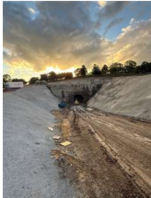
Figure 4. Box-cut and the portal face June 2026.
