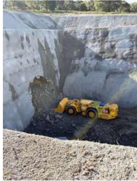
Figure 2. Boggging the first cut from the exploration decline portal.
