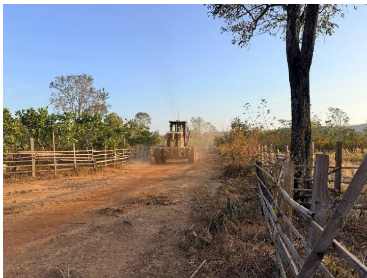
Figure 51| Repair of community road
