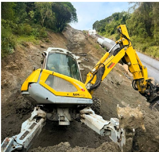
Spider diggers were used for slip stabilisation on the 40-degree slopes beside the Piripaua penstocks.
