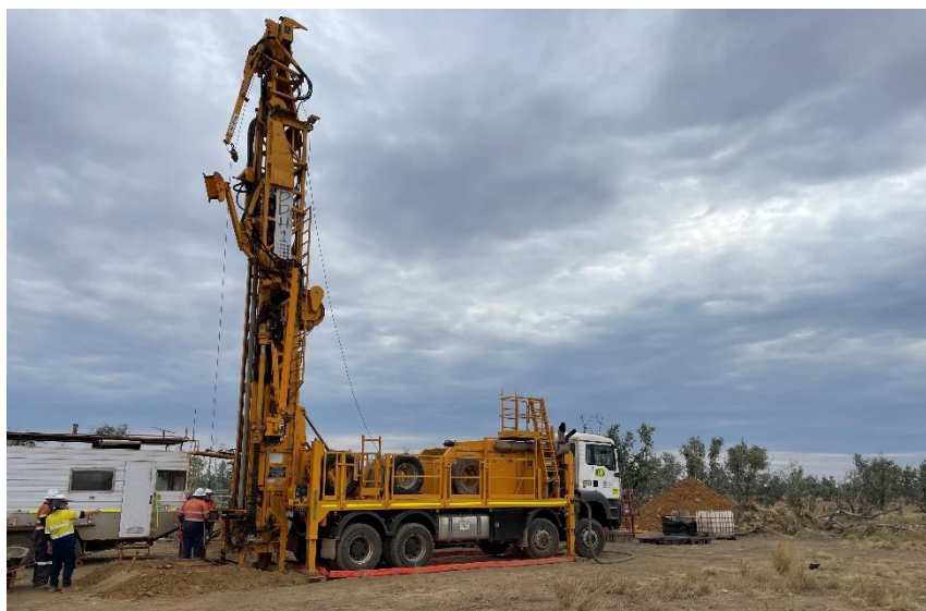
Above: Diamond drill rig onsite testing the Charcoal Bore Prospect at Canobie
