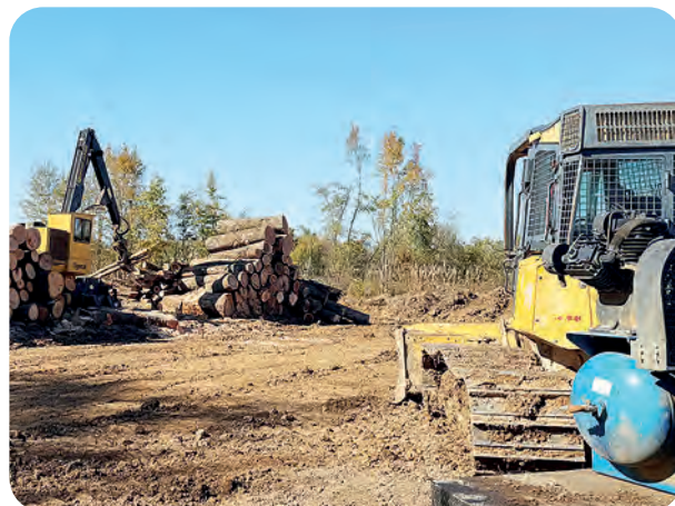
PLEF Site Clearing, Paducah, KY
