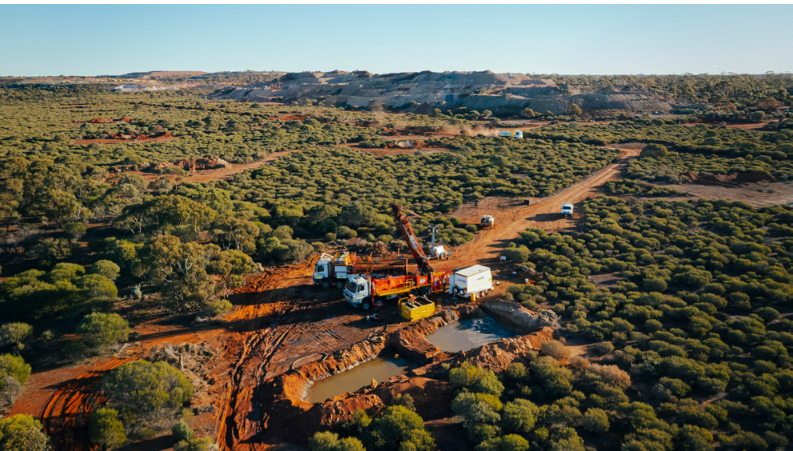
Drill rigs at the Mt Gibson Gold Project.
