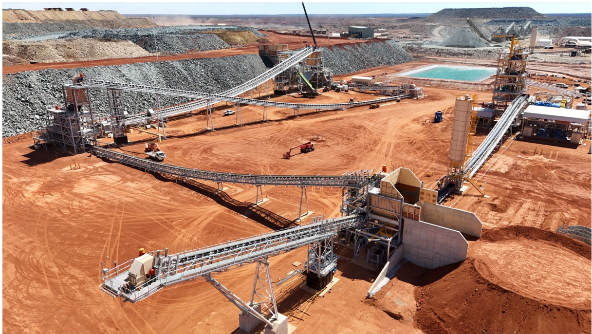
Karlawinda Expansion Project – Surge Bin.
