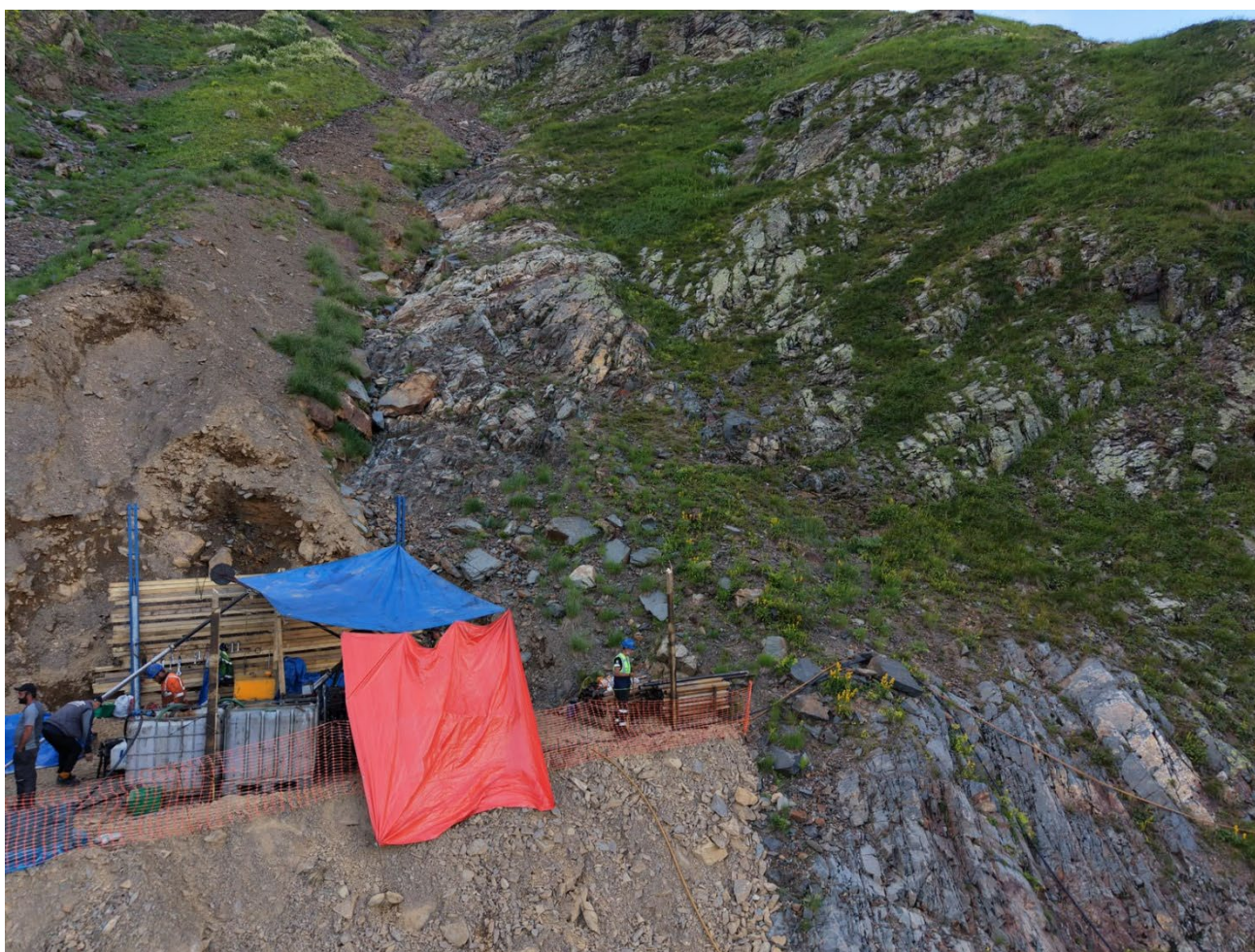
Figure 1 Drill rig positioned on the west flank of the Zopkhito project; location Pad 15
