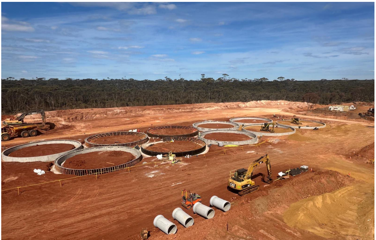
Image 4: CIL Tank Earthworks & Construction underway
