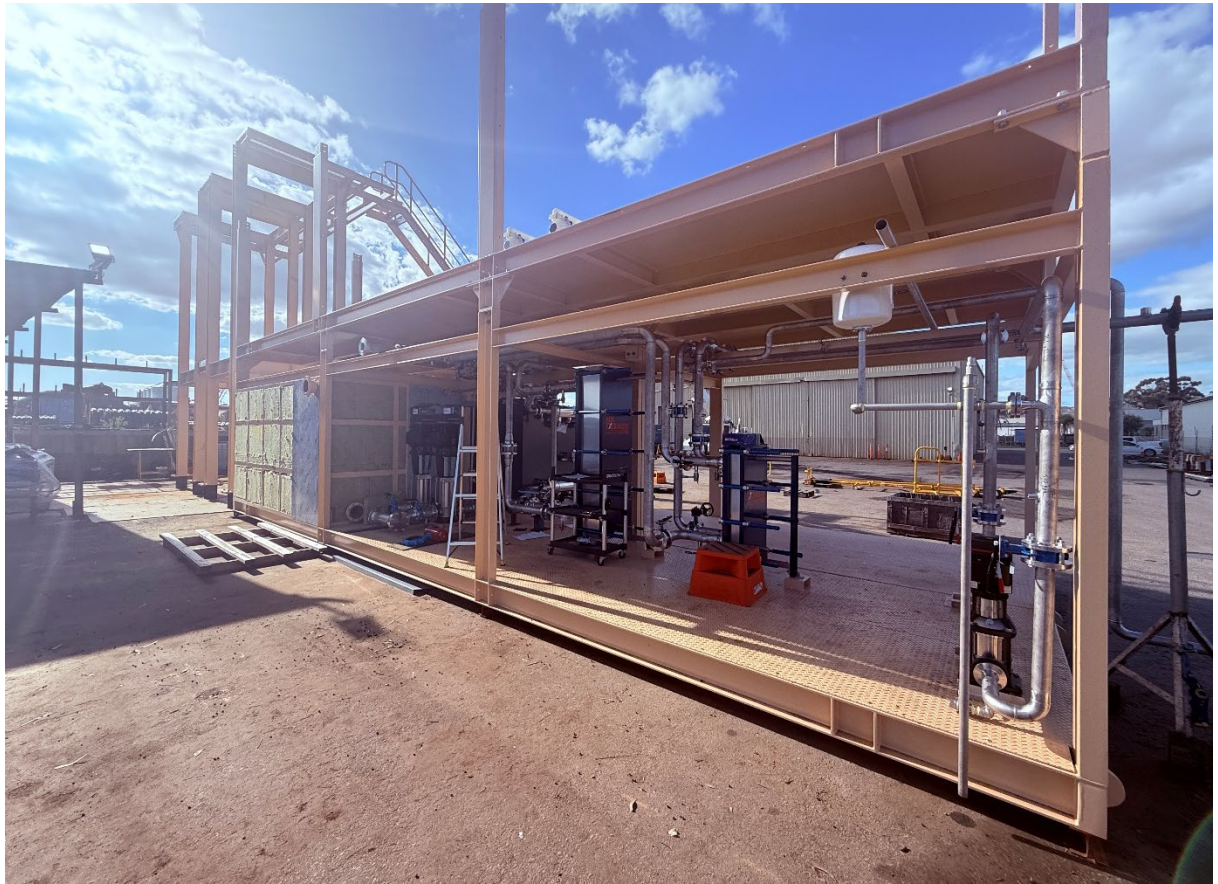
Image 3: Fabrication of Modularised Gold Elution Plant in Maddington, WA
