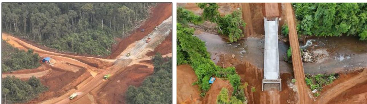
Sampala Mine construction activities
