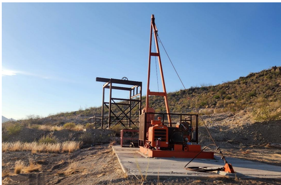
Figure 1 - Shafter Mine hoist repair and refurbishment work ongoing by American Mining and Tunnelling (AMT)
