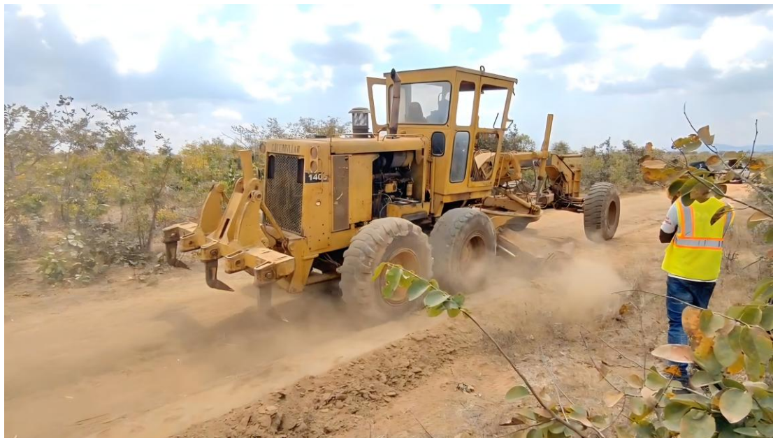
Figure 2: Heavy equipment undertaking road grading works at the Kanyika Niobium Project.
