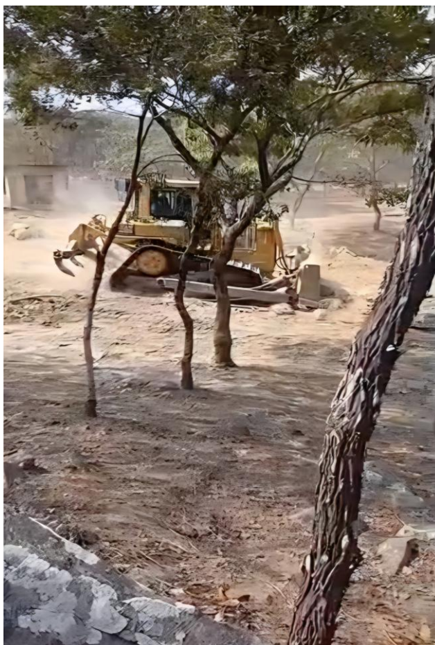
Figure 4: Site preparation and clearing activities underway at Kanyika.
