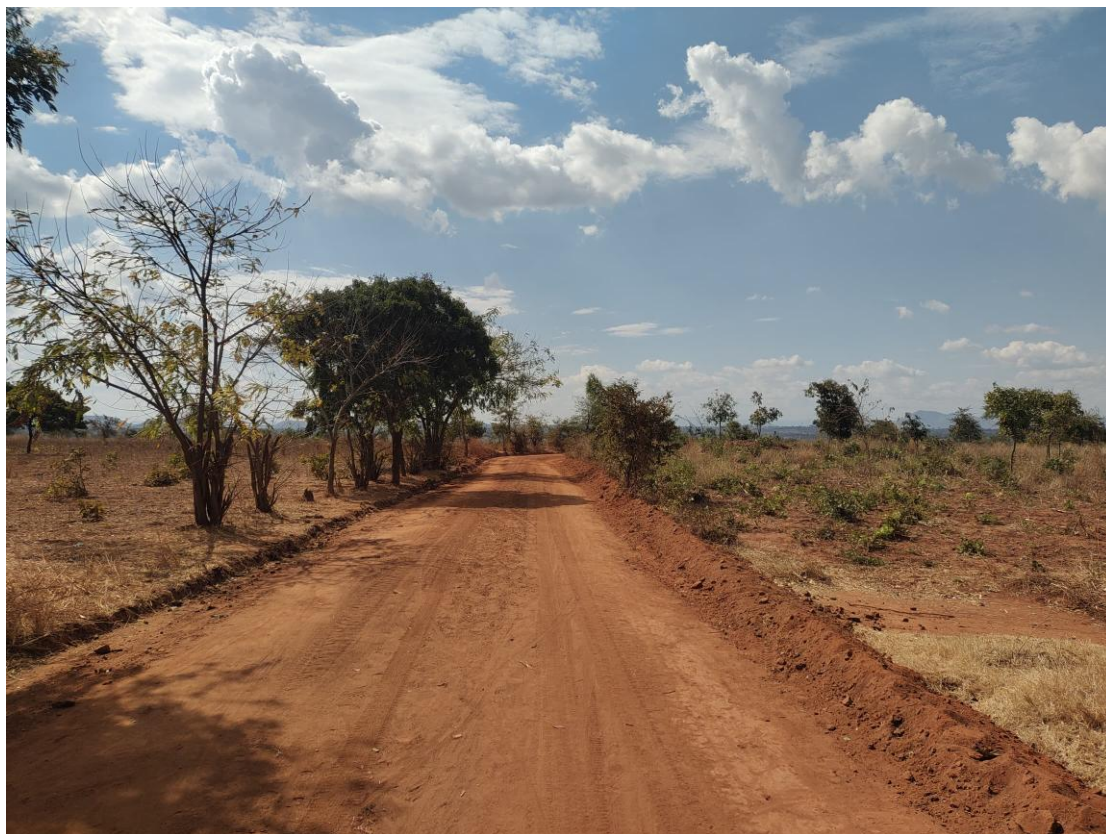
Figure 3: Upgraded section of the main mine access road at Kanyika following grading works.
