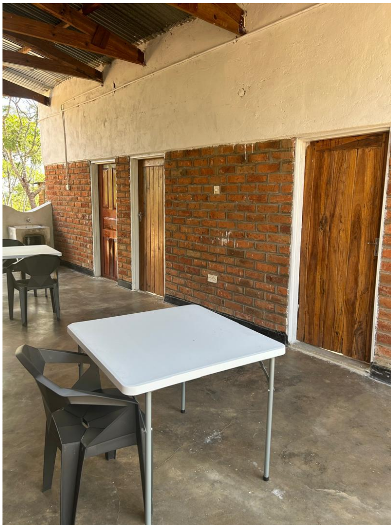
Figure 5: Refurbished accommodation and facilities at the Kanyika exploration camp.
