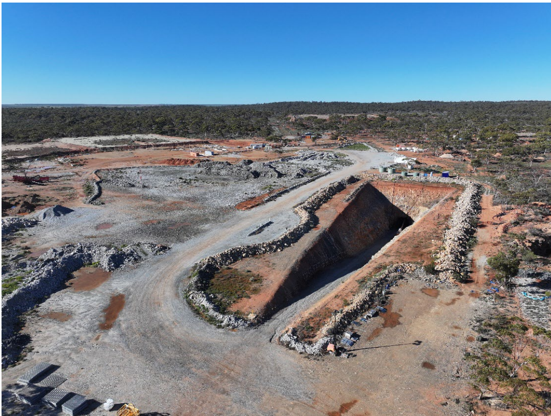
Figure 1: Radio boxcut and portal overlooking the proposed ROM and processing area
