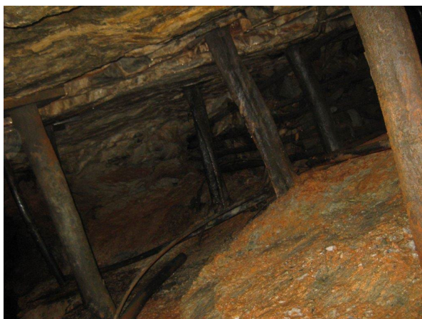
Figure 10: Historical Radio underground workings (Level 9)
