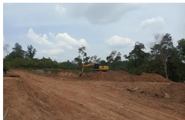
Initial site preparation and earthworks
