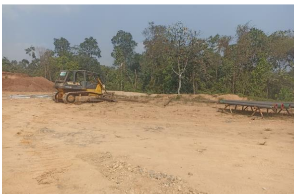
Site leveling activity
