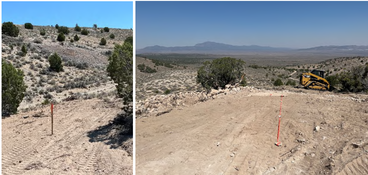
Figure 2- Drill pad preparations- North Star Prospect
