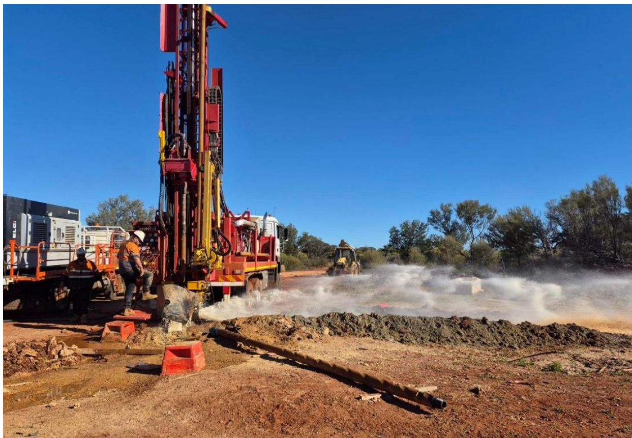
Figure 1: Water bore drilling Mulgabbie North
