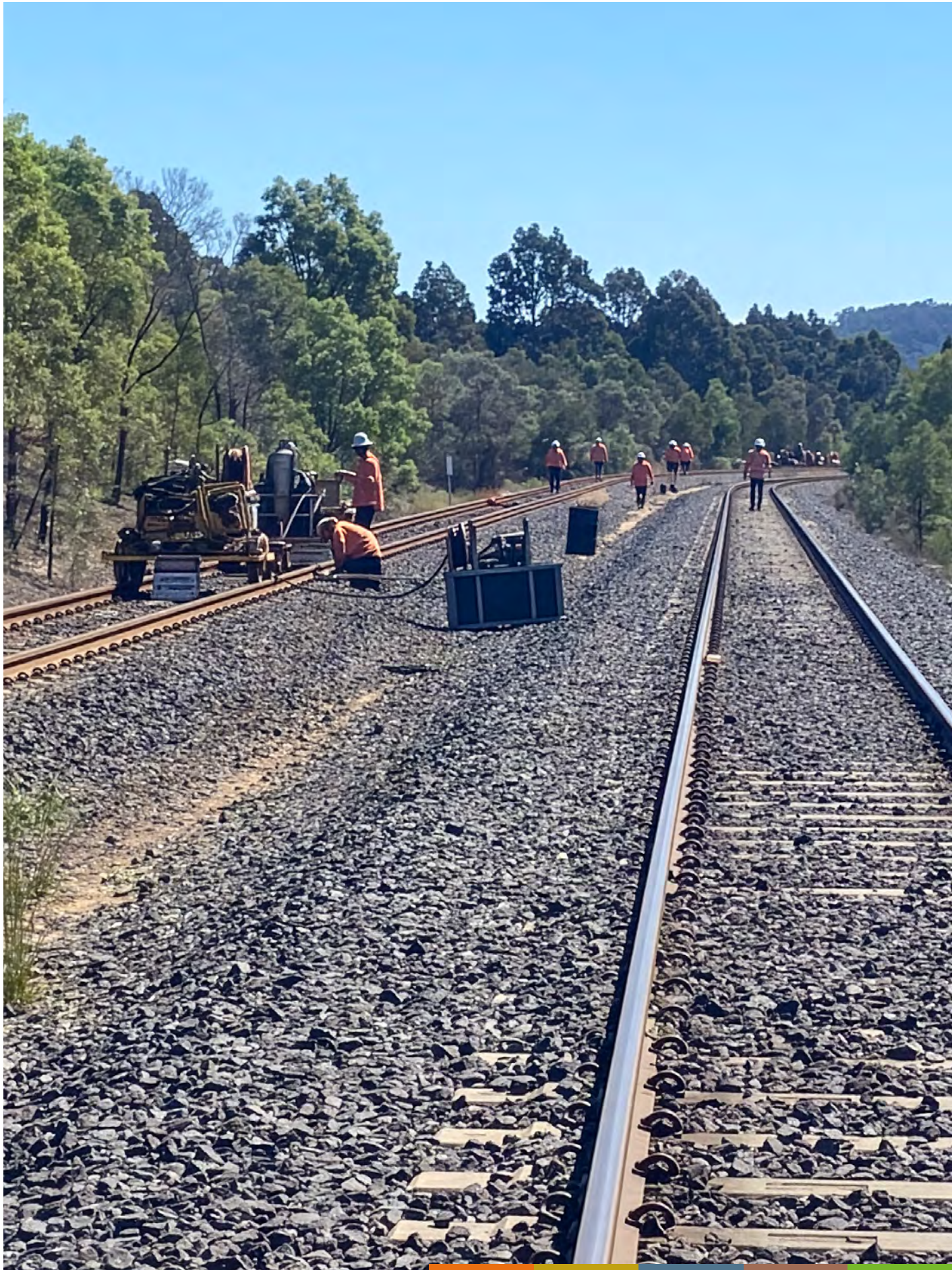
Wilpinjong Rerailing Project, New South Wales
