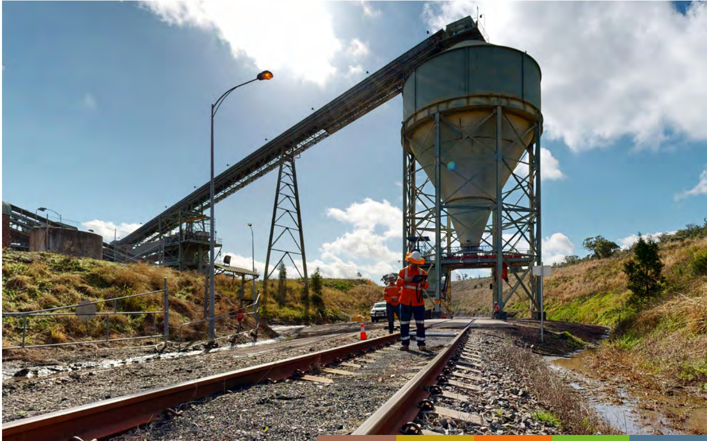
Track inspection, New South Wales
