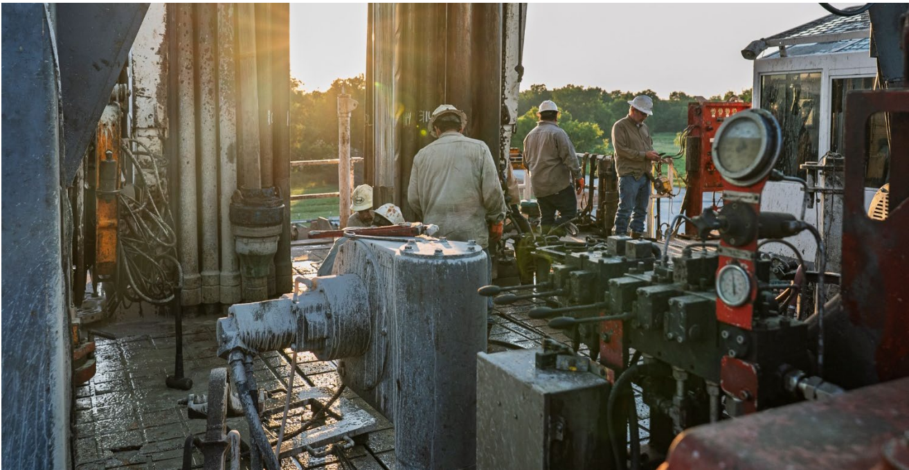
Kenai Drilling Rig 18 on the Suttles pad in the SWISH AOI, Oklahoma.
