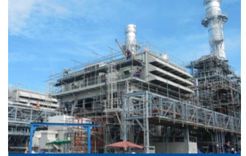
Heating & Cooling Systems
