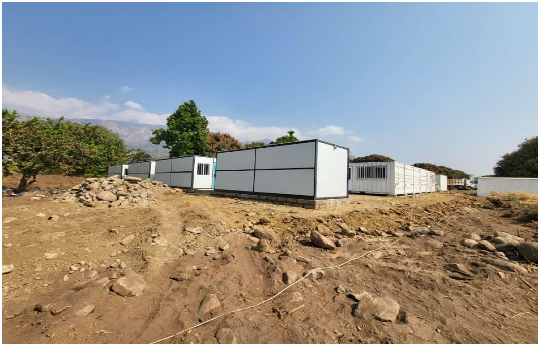
Image 2: Camp construction is complete, with commissioning activities now underway.
