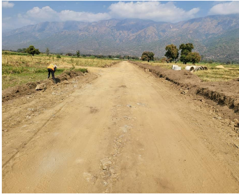
Image 1: The newly constructed access road to Kinambo-2 is now complete and ready for operational traffic.
