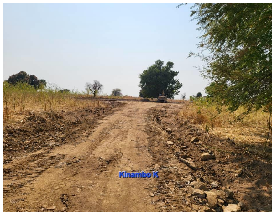
Image 3: The Kinambo well pad taking shape ahead of the drilling rig's arrival.
