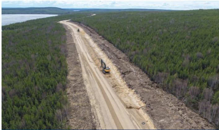
On-site Access Road
