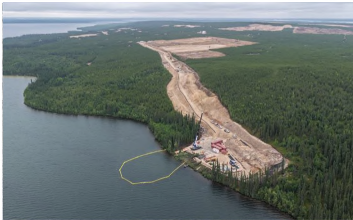
Diffuser Installation and Access Road
