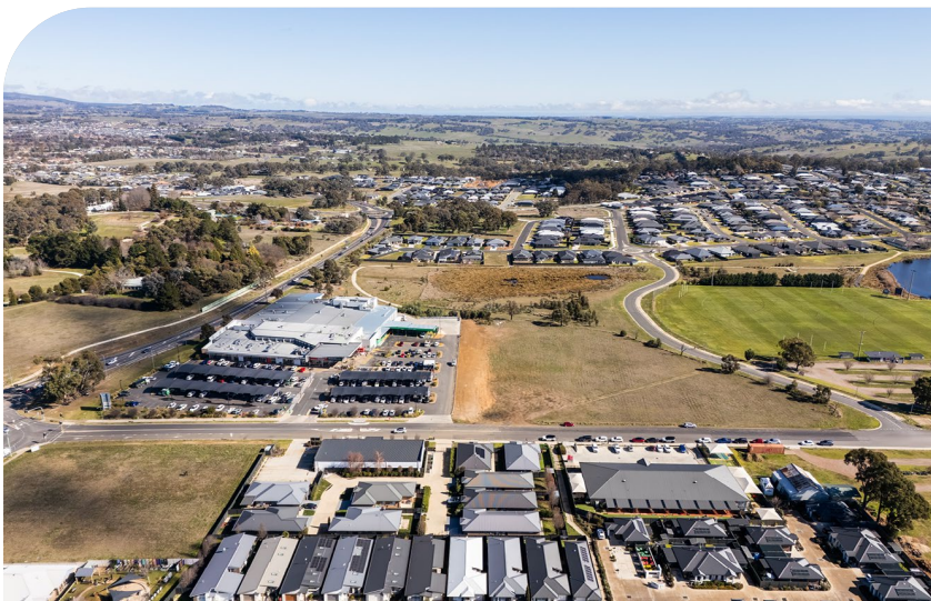
North Orange Shopping Centre, NSW
