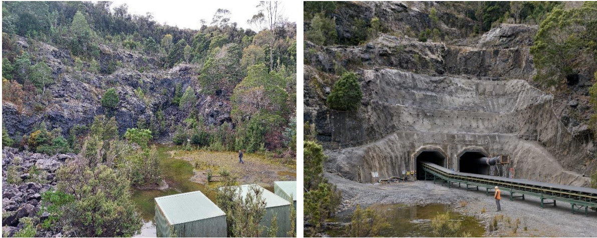
Figure 3: Existing HEC Quarry area proposed for the Mt Lindsay underground mine portal (left), together with an illustrative underground portal arrangement (right). Locating the principal mine access within the existing quarry disturbance is being evaluated as part of the Scoping Study, with the objective of reducing the requirement for new surface disturbance. Final portal location and configuration remain subject to ongoing engineering, environmental assessment and regulatory approvals.
