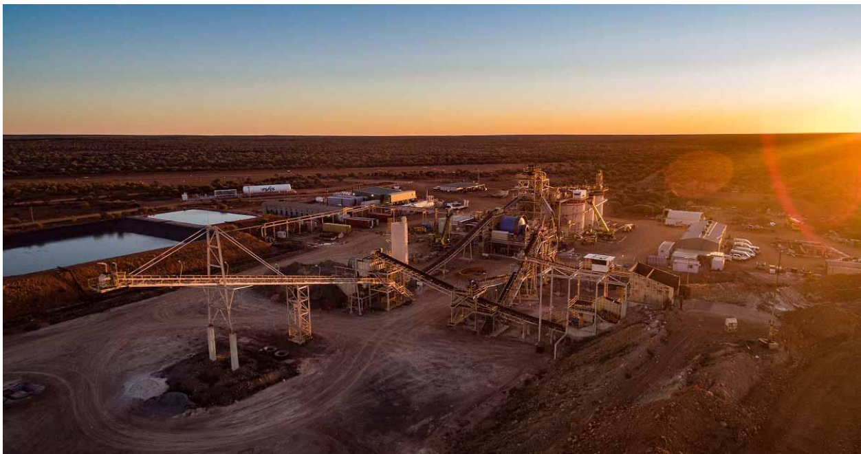
Figure 1: Kirkalocka Processing Facility 2026
