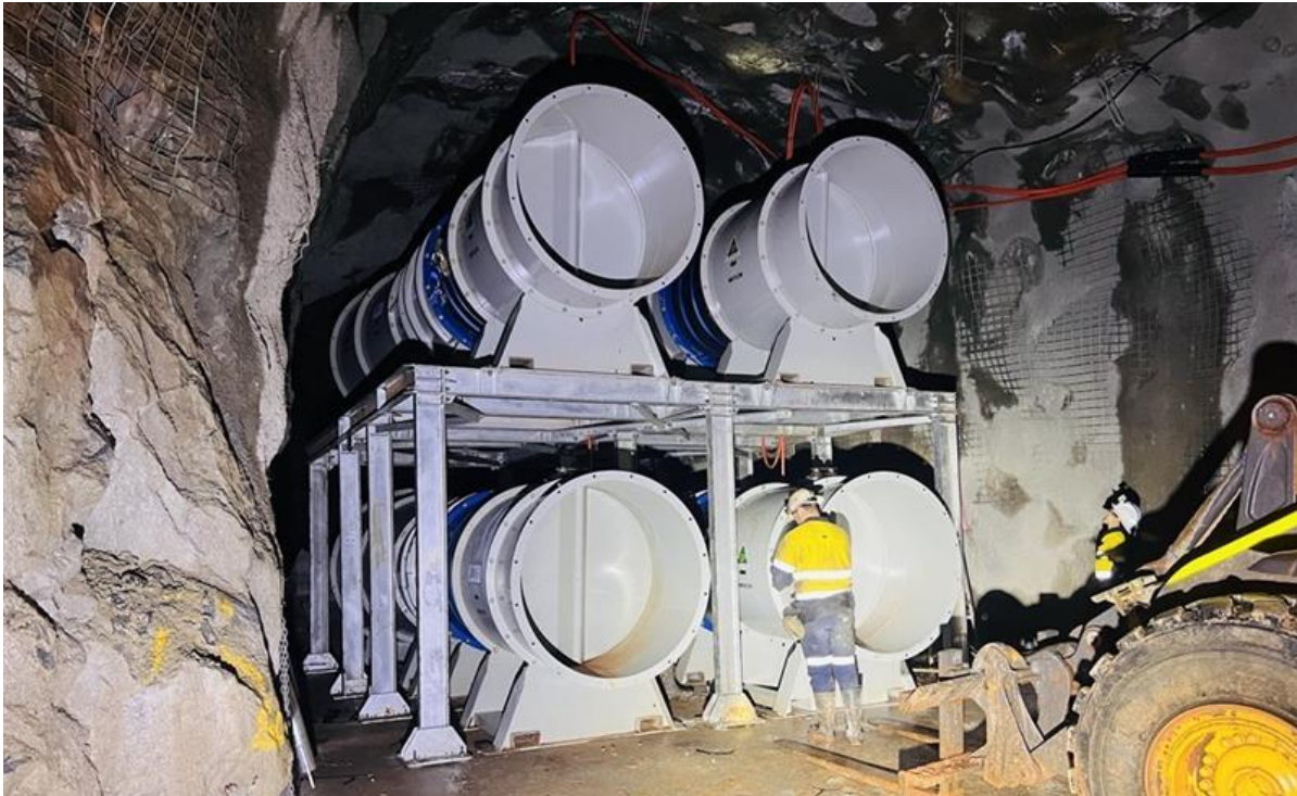
Figure 9 – Installing primary ventilation fans in United North
