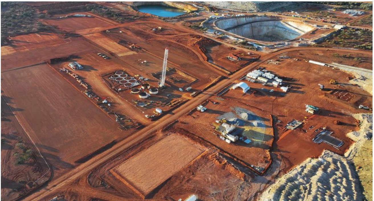
Figure 7 – Mill construction at Youanmi
