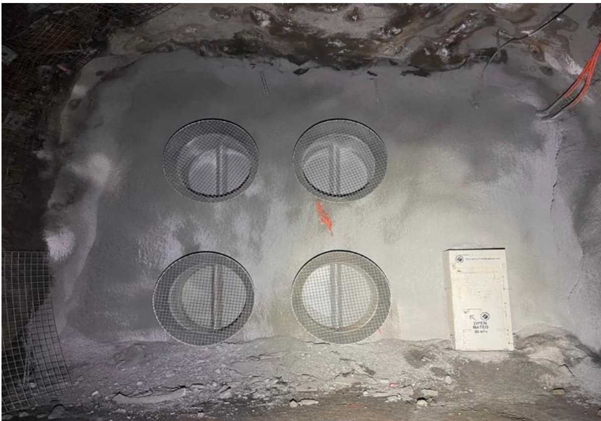
Figure 10 – Installing primary ventilation fans in United North
