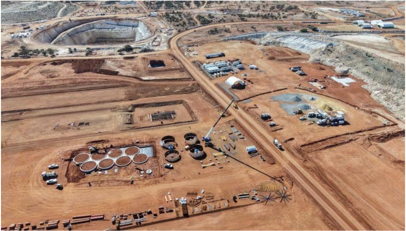
Figure 6 – Progress of construction on site
