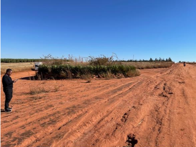
Figure 2 – Existing Regional Road – Undeveloped
