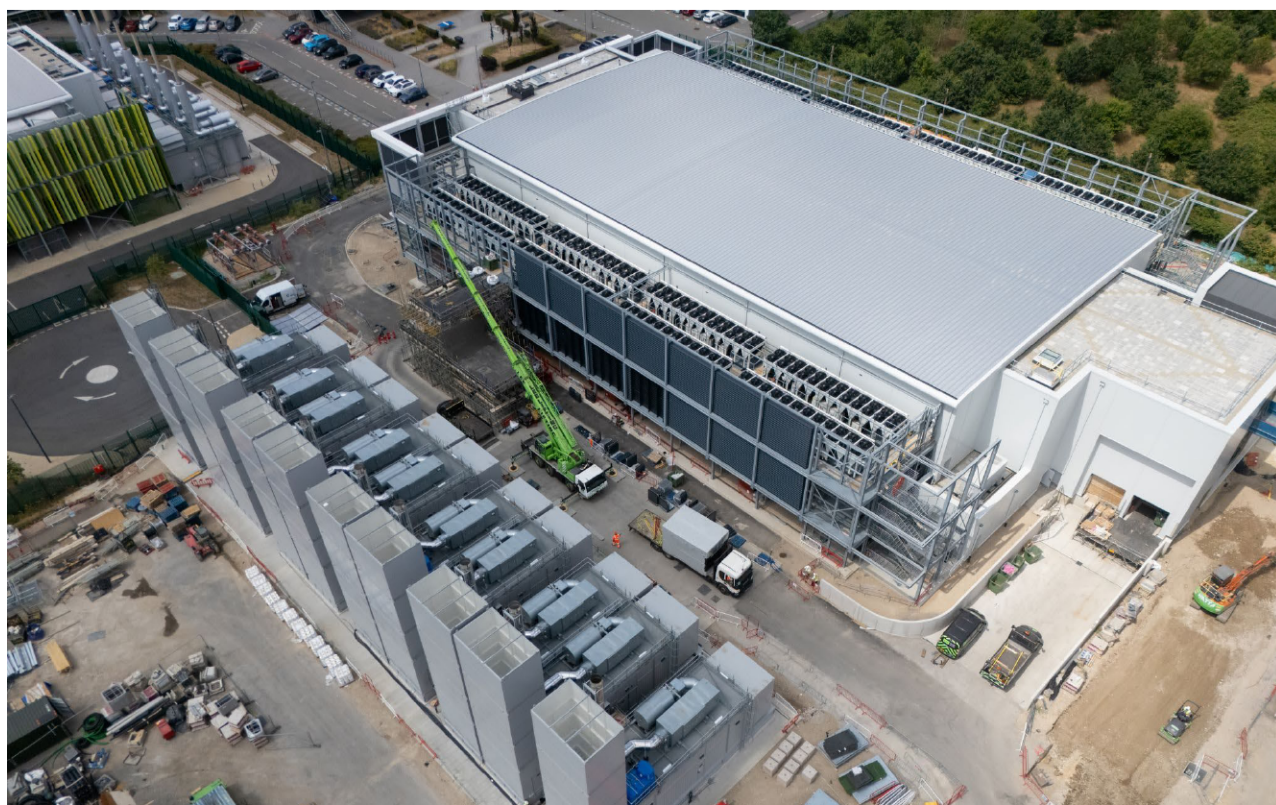
Construction underway at Kao’s KLON-03 facility
