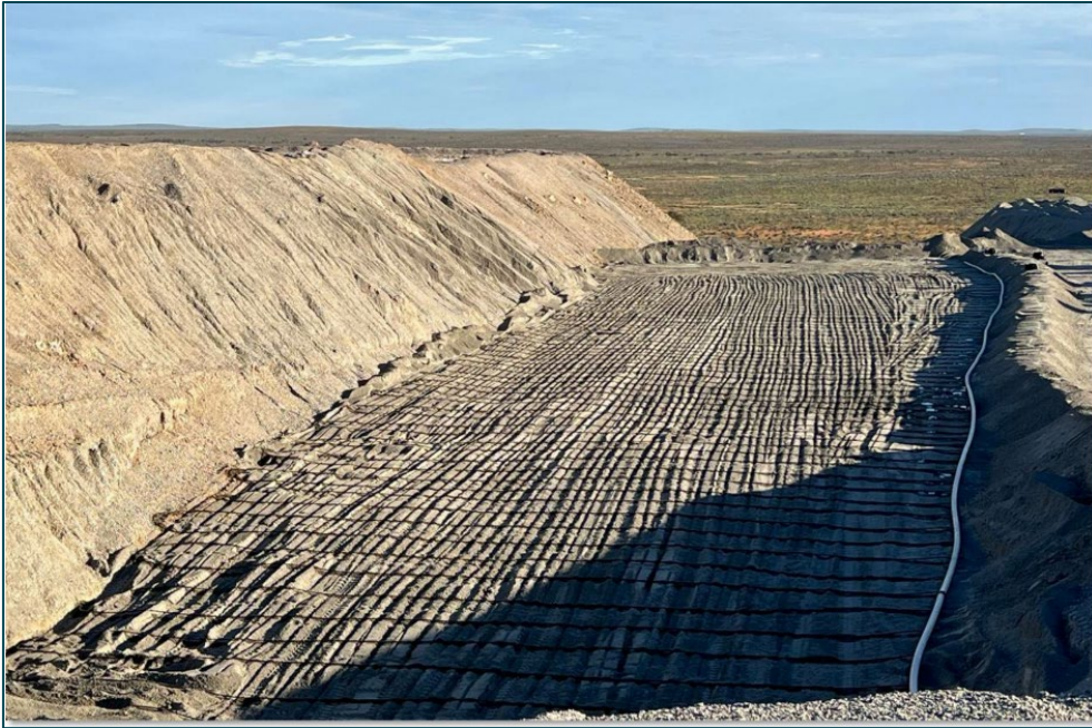
Photo 1: First re-crushed heap leach material now under irrigation
