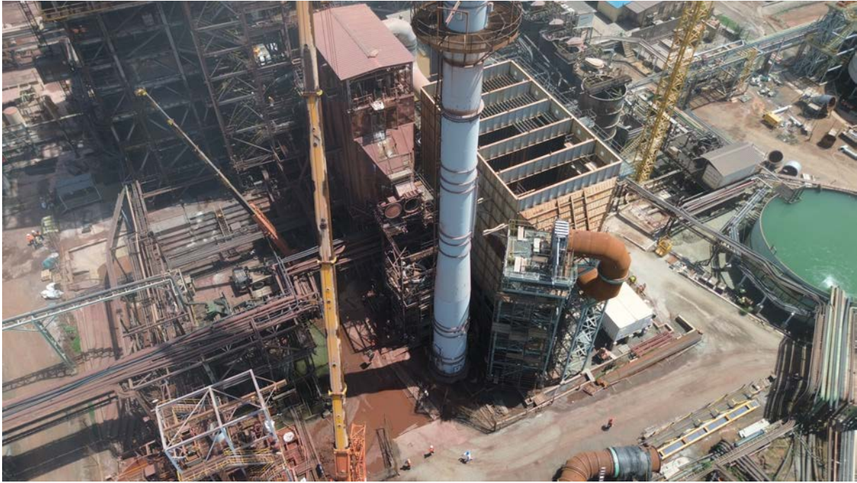
Figure 8: New Electrostatic Precipitator being tied in
