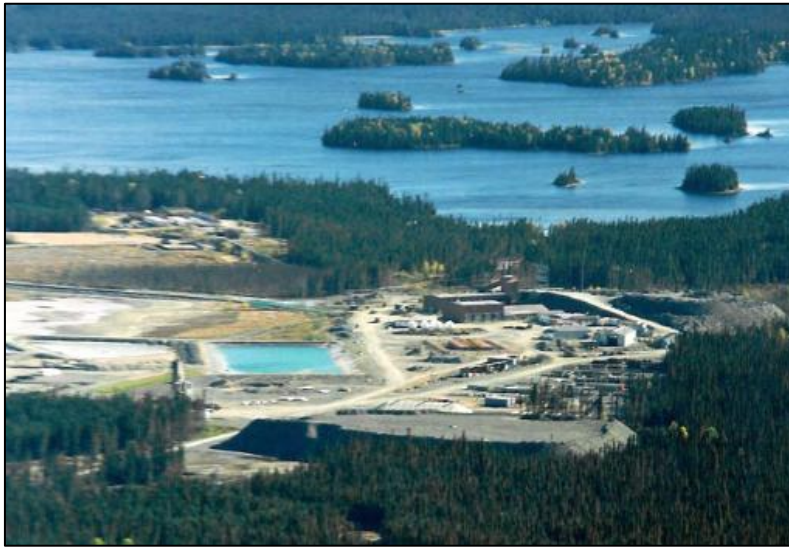
Figure 5 - Golden Patricia Gold Mine. Active operations in foreground looking east, circa 1996
