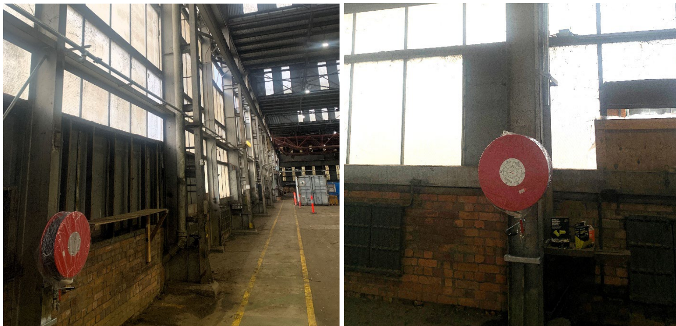
Fire protection installation progress with new fire service piping and hose reels installed
