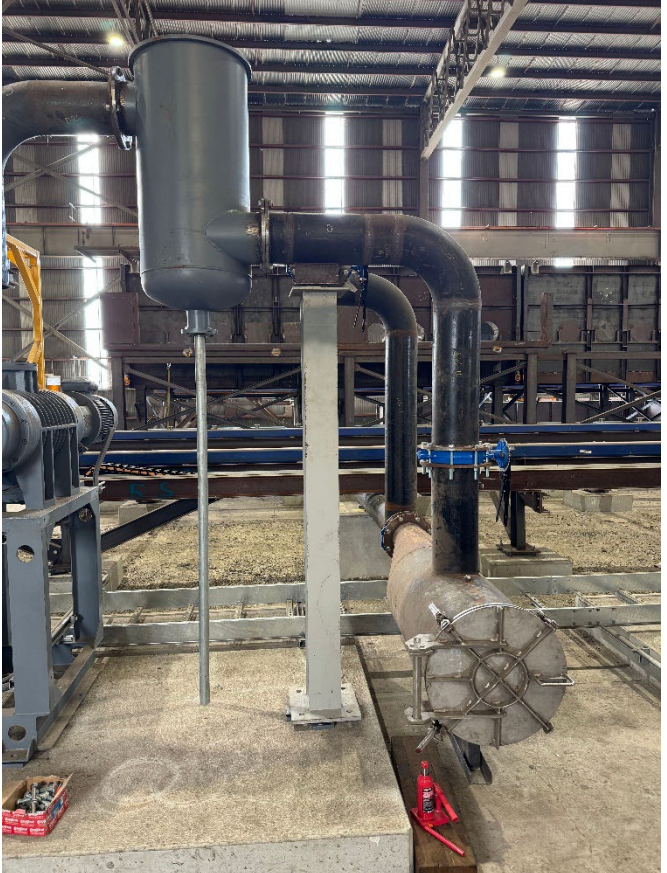
Vacuum piping manifold fabrication and piping installation, along with Baler installation progress
