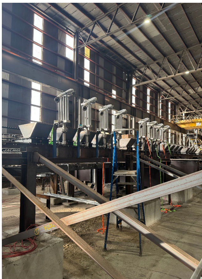
Ducting and reagent piping and Reduction Furnace vacuum Special Piping item installation progress
