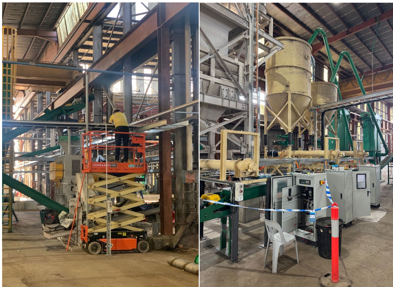
Briquetting terminations complete and initial pre-testing of electrical equipment
