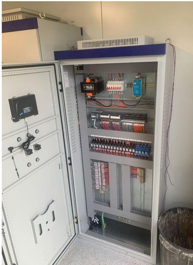
Briquetting substation wiring modifications, electrical and instrumentation cable installations for Briquetting, Baler, and Refinery installed
