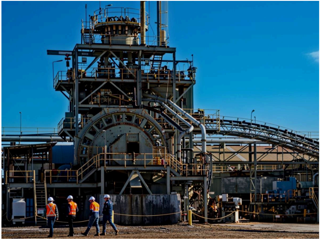
Figure 2: Edna May Processing Facility
