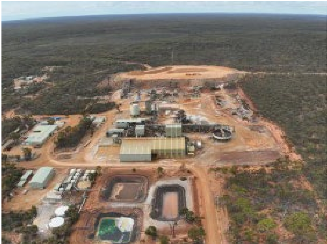
Figure 3: Lake Johnston Processing Facility
